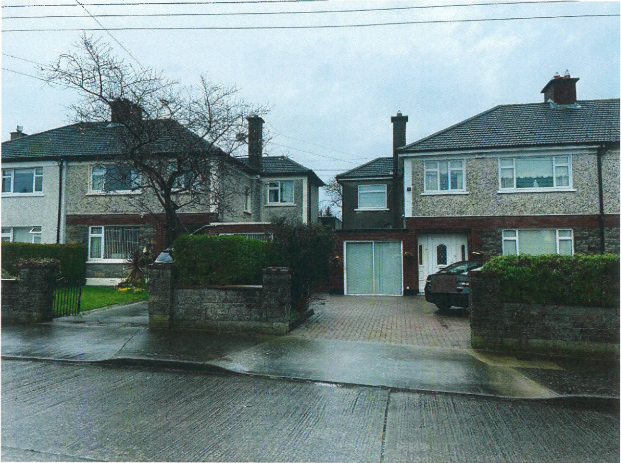
Photo No. 7: Nos. 17 (LHS) and 18 (RHS) – both have converted the garage but with different window treatment/elevation treatments and at first floor level both are different with pebble dash at No. 17 and bare concrete render at No. 18.
