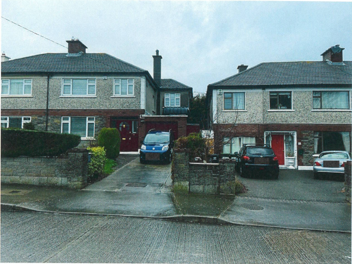
Photo No. 3: No. 21 on the LHS has added a porch door and also has a non-painted render finish to the walls above the garage plus there is a fuel tank on the roof of the garage. No. 22 on the RHS has converted the garage and extended at first floor level above the garage. The new/additional pebble dash at first floor level is different in colour and appearance to the older pebble dash – it is brighter like our client's at No. 16.
