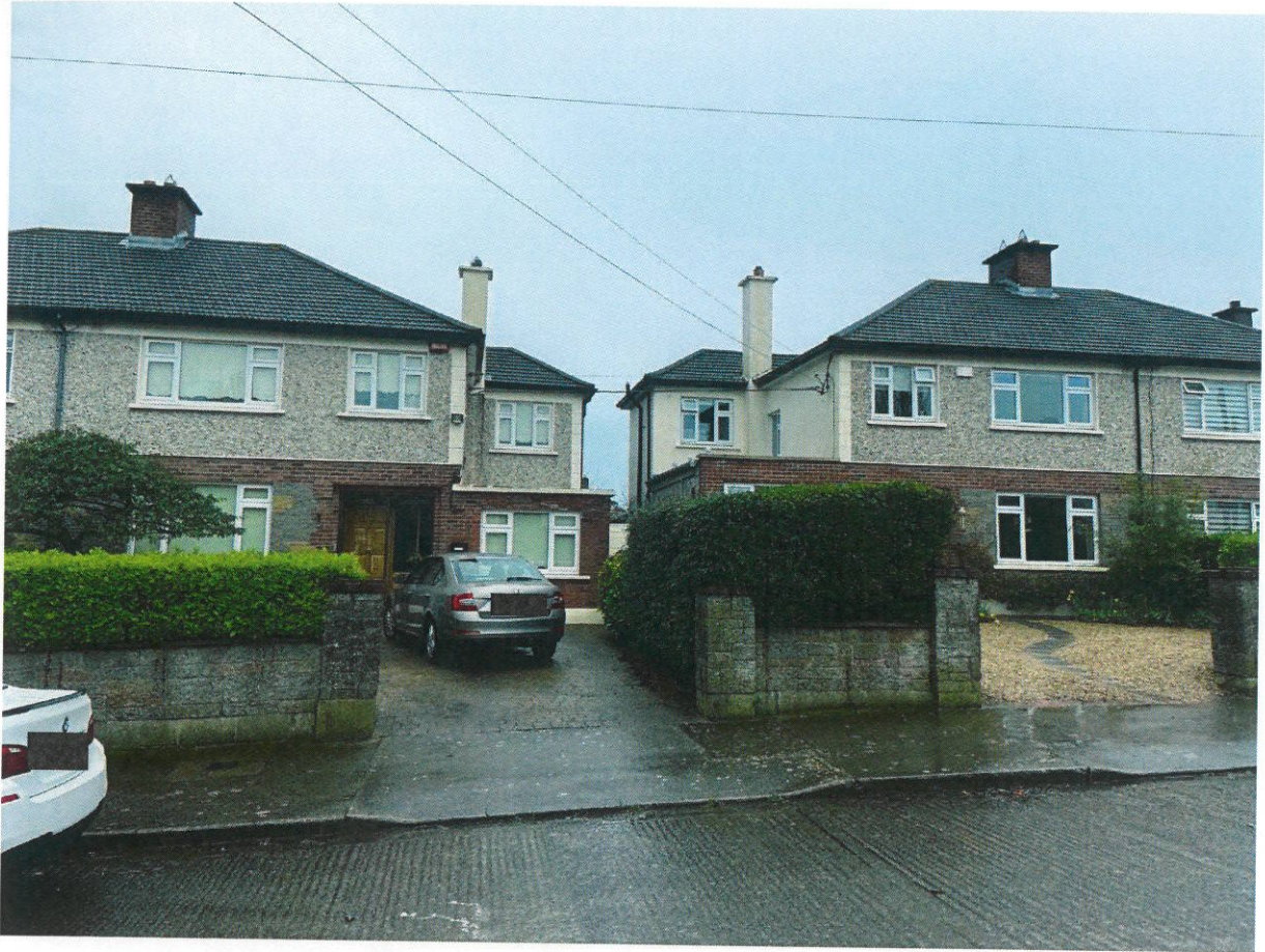
Photo No. 5: These are Nos. 4 and 5 and both have converted the garage but both also use different finishes at first floor level – pebble dash and painted render.
