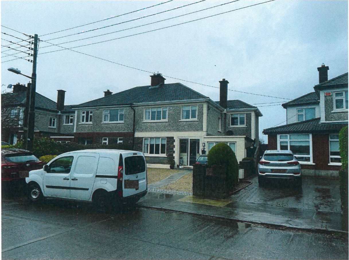
Photo No. 2: [REDACTED] (on the left hand side - LHS) has painted over the brickwork, added a sliding porch door and changed all the windows. No. 26 to the right hand side (RHS) has converted the garage, added a pitched roof and has a painted render finish at first floor level.
