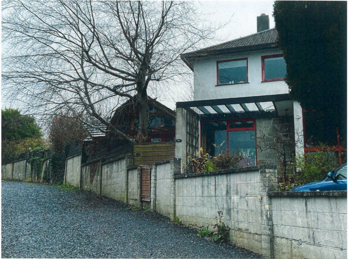
Photo No. 11: This appears to be a two storey timber structure within the side garden of No. 11.
