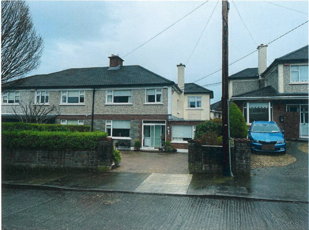
Photo No. 4: No. 1 on the far LHS has extended above the garage; No. 2 in the centre has converted the garage and painted the concrete render wall above the garage, whereas No. 3 on the RHS has converted the garage with a bay window, added a pitched roof and omitted a first floor window.
